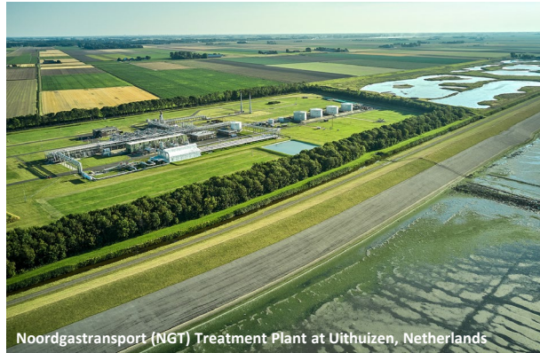
Noordgastransport (NGT) Treatment Plant at Uithuizen, Netherlands
